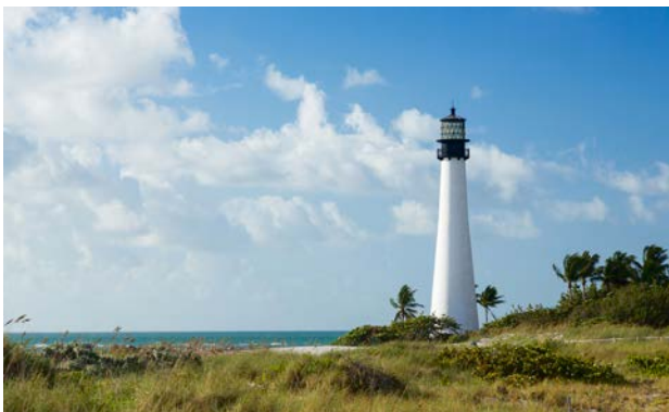
Cape Florida Lighthouse
