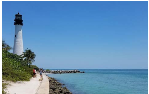
Seawall along lighthouse promenade
