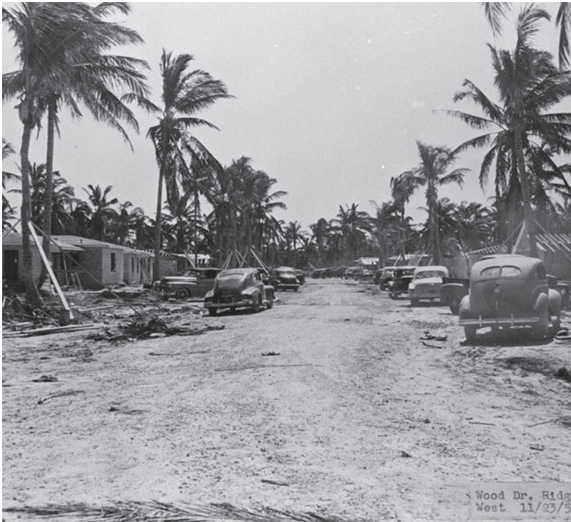
Construction of the Mackle Homes on W. Wood and Ridgewood (1950). Source: https://www.kbhistory.org/page/3/ .
