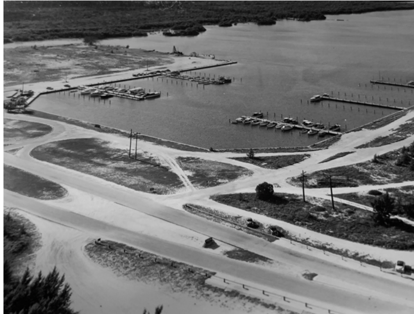
Crandon Park Marina under construction (1953).
