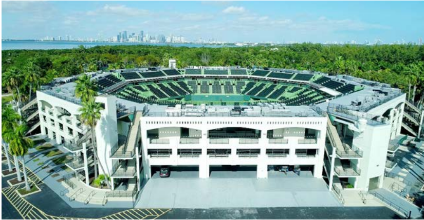
Tennis Stadium exterior/interior in good condition
