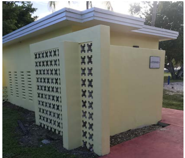
Storage with ornaments of the South Florida Vernacular Architectural Style
