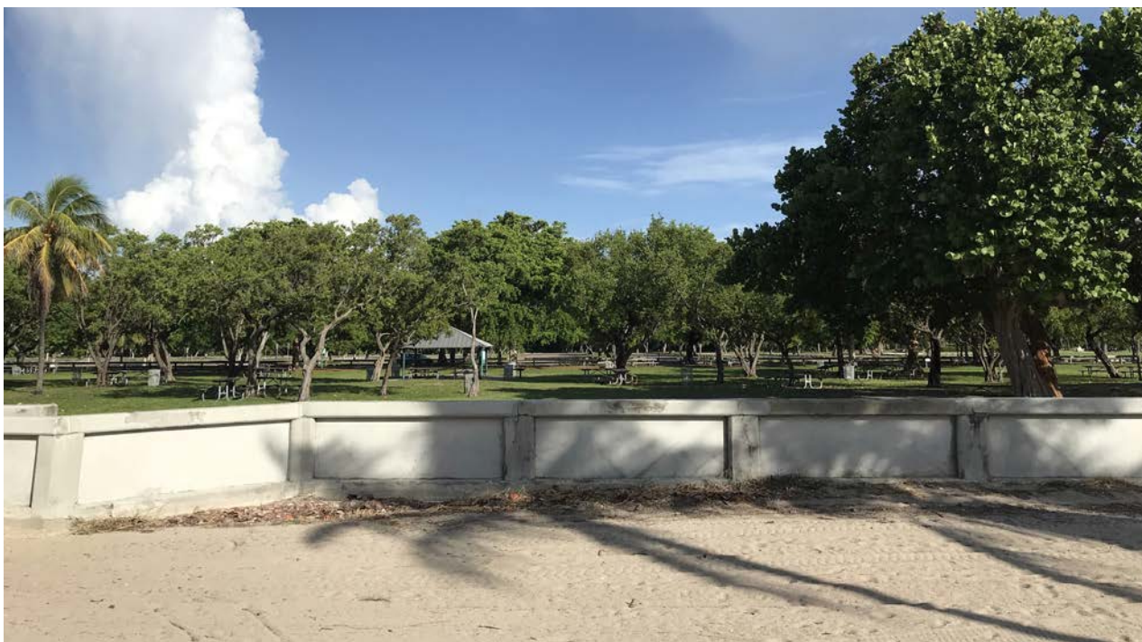
Beach sand wall acts as a blockage and restricts access from beach to the picnic grounds and vice versa
