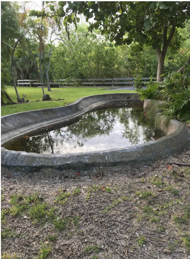
Concrete-lined former zoo pond
