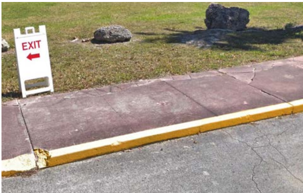
Cracked sidewalk
