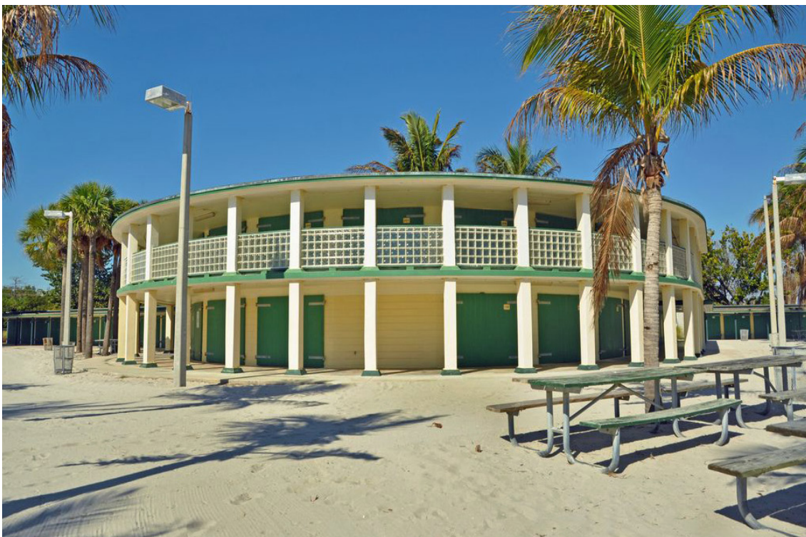
Circular cabana appear in overall good condition
