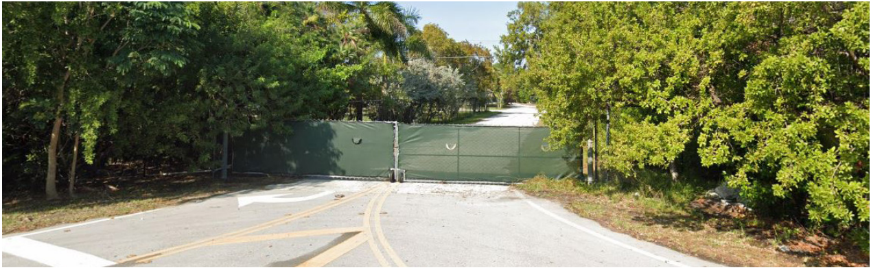
Blocked entry at Tennis Center North Entry
