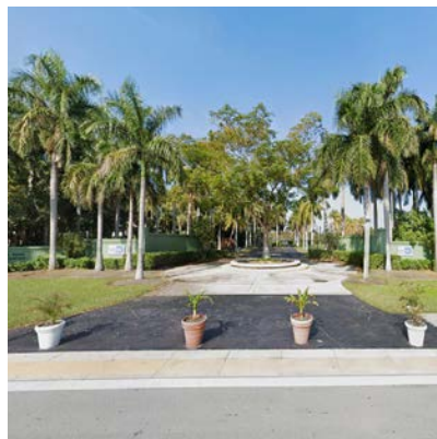
Main Entry now used for pedestrians is a remnant of previous vehicular access.
