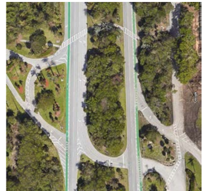
Bike/Pedestrian Crosswalk at Golf Course
