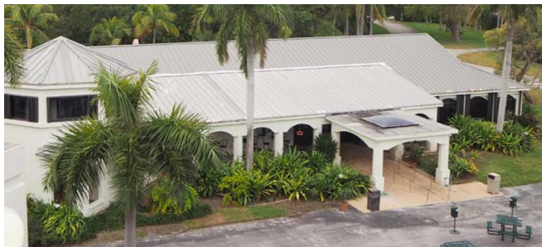
Tennis Clubhouse exterior is in good although interior in poor condition
