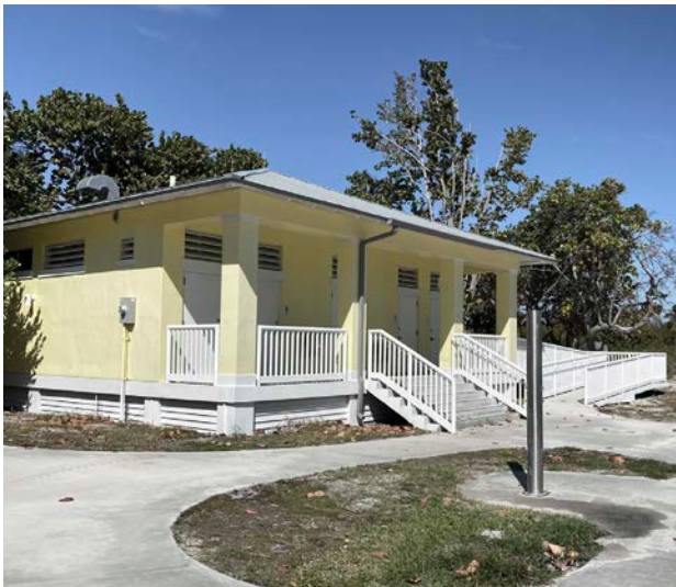
Restrooms with ADA access
