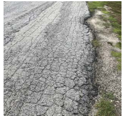
Cracked asphalt
