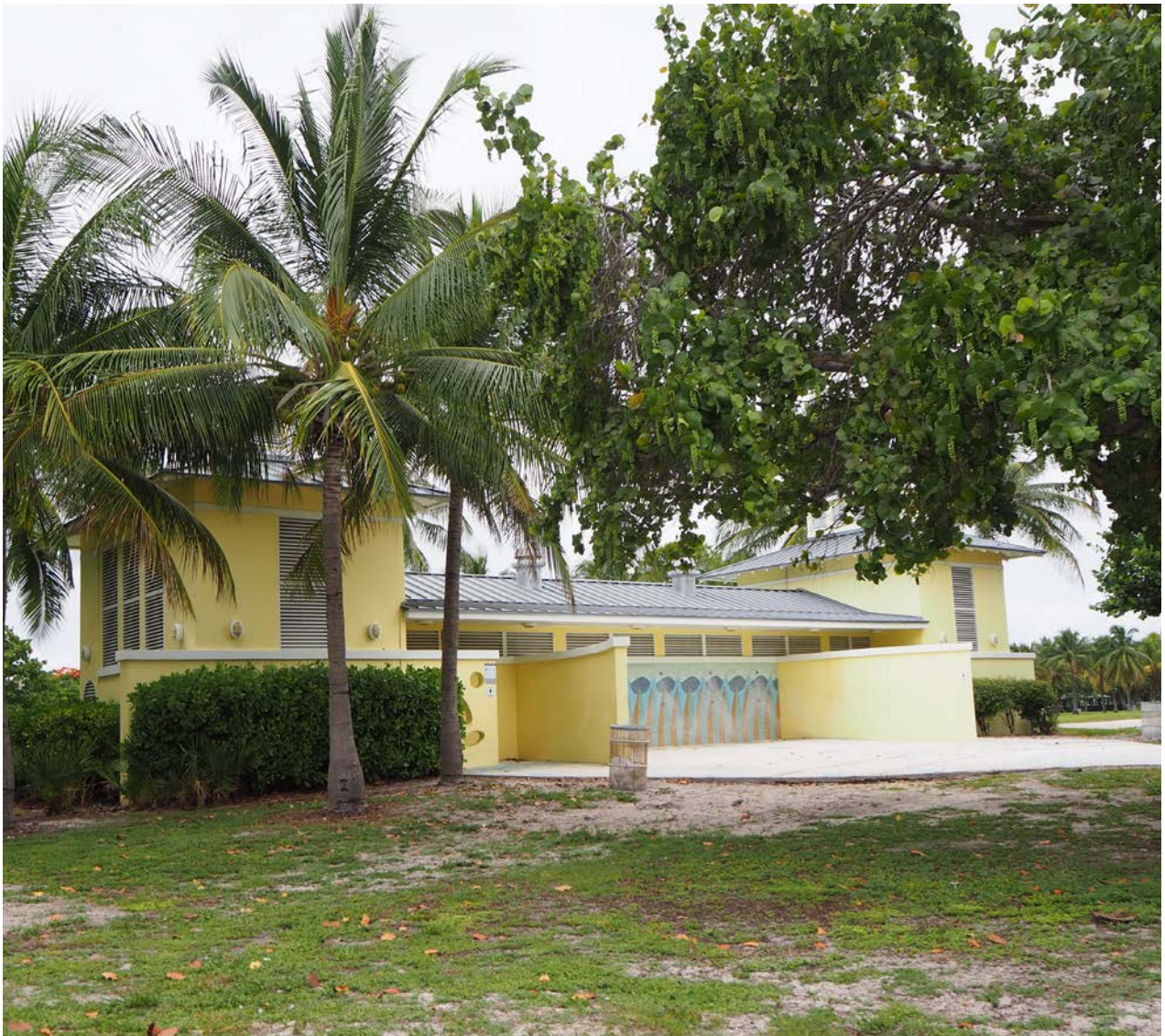
Restrooms and showers are generally in good condition
