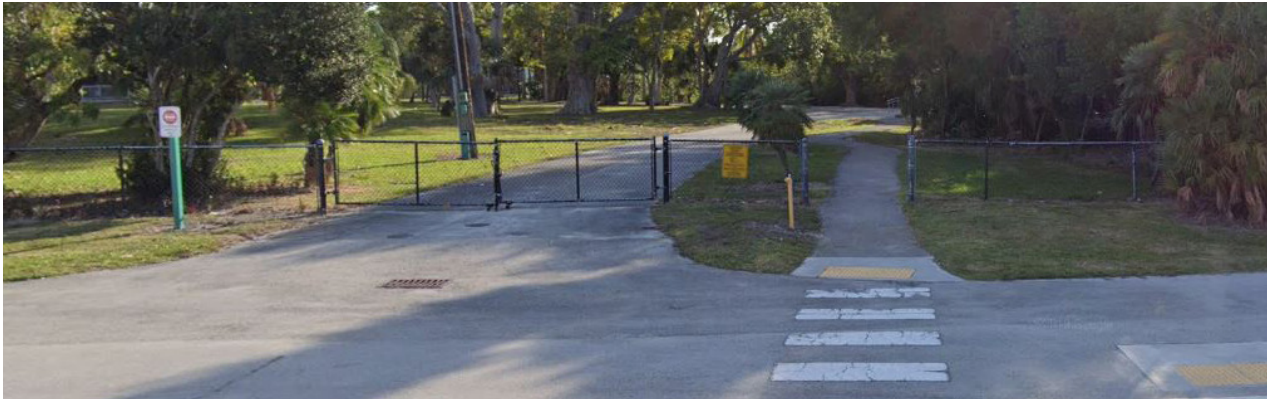
Uninviting entrance to Crandon Gardens from North Parking Lot West side
