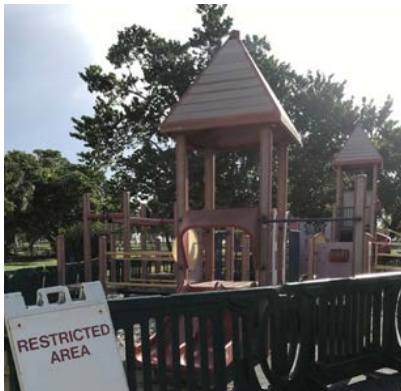
Play equipment in poor condition
