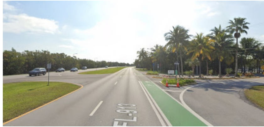
Marina Entry - lacks welcome grand arrival experience and clear entrance mark. Also signage is too small for drivers to recognize an entrance on time
