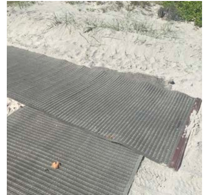
The only ADA path to the Beach in poor condition
