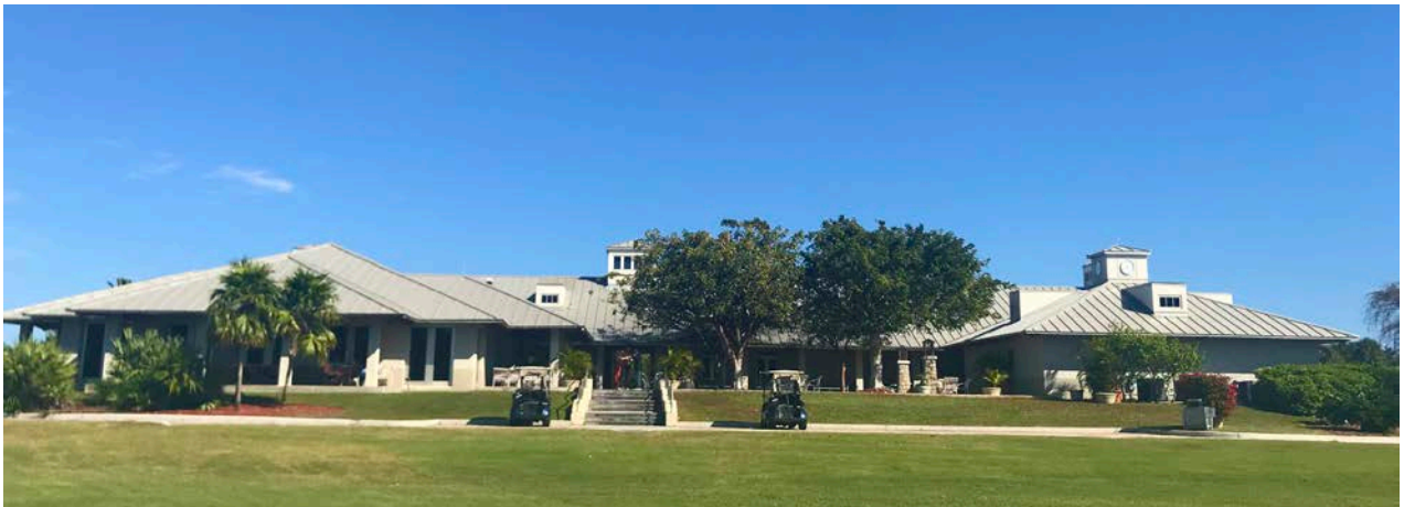
Golf Clubhouse is in fair condition, but out-dated
