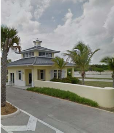
Park offices in good condition, level of use unknown
