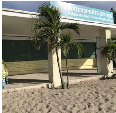
Watersports Center in fair condition
