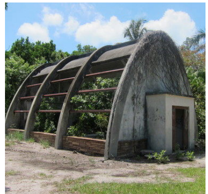
Abandoned zoo structure
