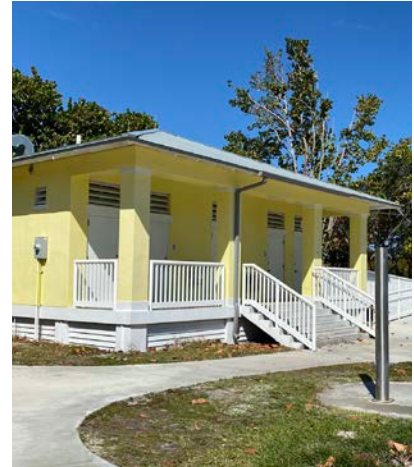
Beach restroom facilities are in good condition
