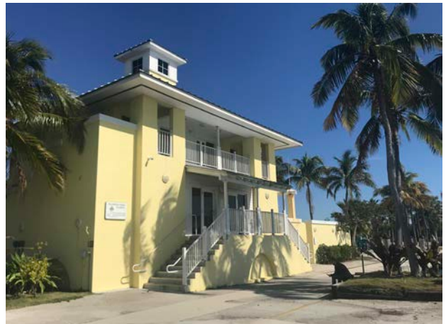
Marina facilities are in good condition, but out-dated
