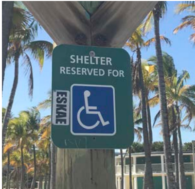
ADA signage in good condition
