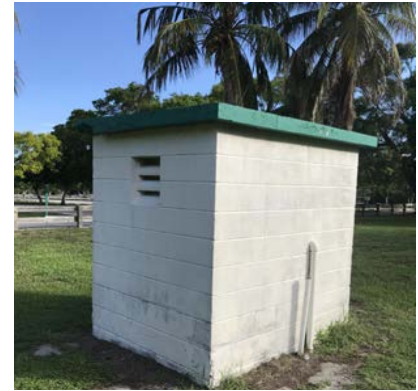
Various unknown structures scattered throughout the site
