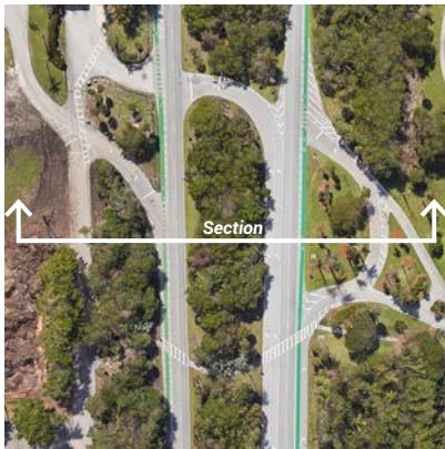
Golf Course Entry aerial view
