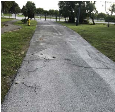
Damaged path in Crandon Gardens
