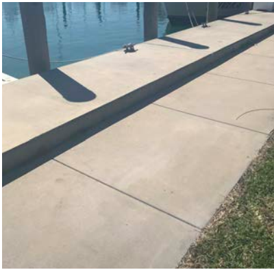
Sidewalk along Marina water in good condition
