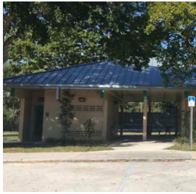
Restroom structure at Calusa park in good condition
