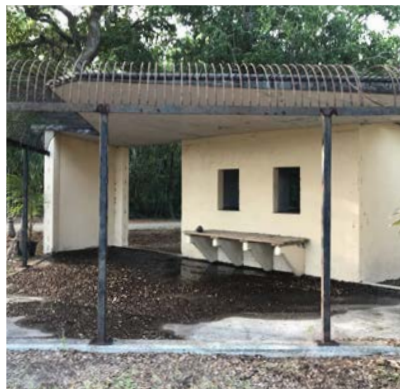
Abandoned zoo structure
