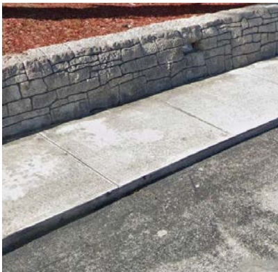
Sidewalk to Golf Clubhouse in fair condition
