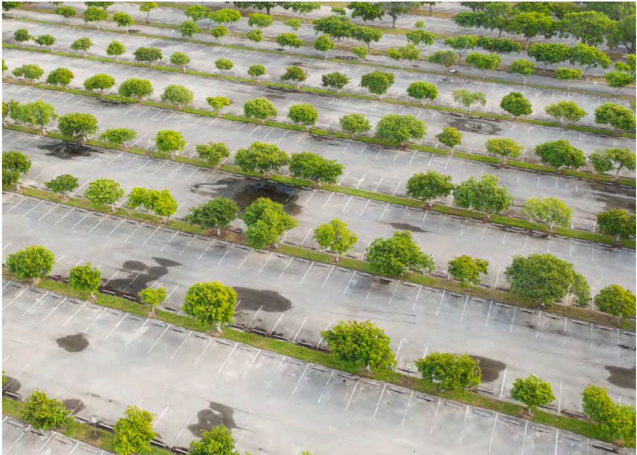
Crandon Park is overly car-oriented. Empty asphalt parking lots cover valuable upland. On-site observation suggests that the parking capacity exceeds current visitorship.
